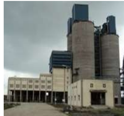
Cement Silo(cap:2X10K, 1X5K)
